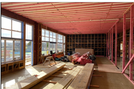
The classrooms will be opened up but there will also be doors between each room to either open up the entire space or close off each room. There will be new lighting and new acoustic ceiling panels and the walls will be lined with Autex to reduce noise.
